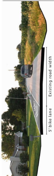
Section cut through Jackson Boulevard showing 5' wide bike lane (looking north)
